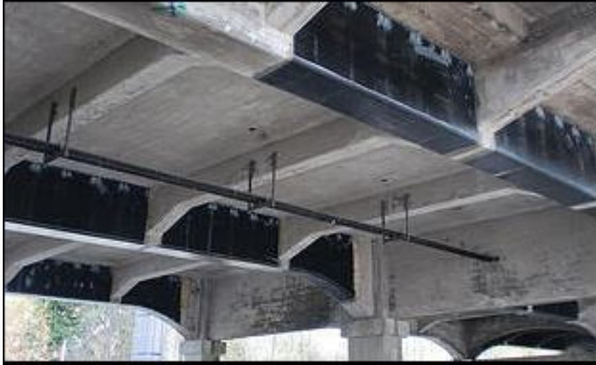
Figure 1.4: Reinforcement of concrete bridge using carbon fibres.
