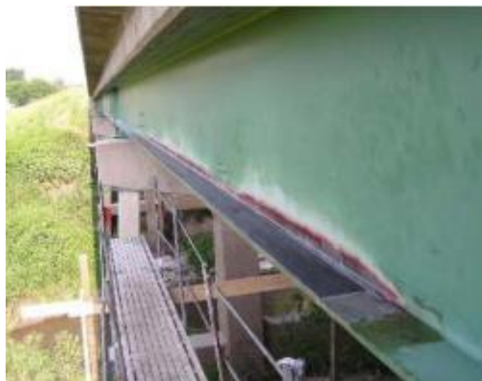
Figure 1.20: Prefabricated pultruded carbon strips bonded onto a steel bridge.
