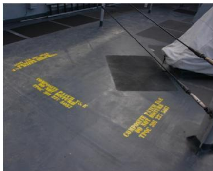
Figure 1.11: Glass fibre patching of sensitized aluminium deck.
