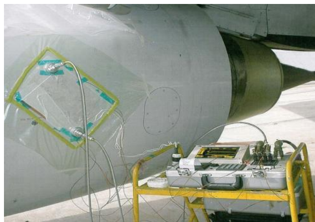
Figure 1.21: Curing of co-bonded patch.
