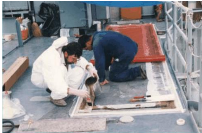
Figure 1.2: Application of a composite patch on site ( Grabovac et al, 2009 ).
