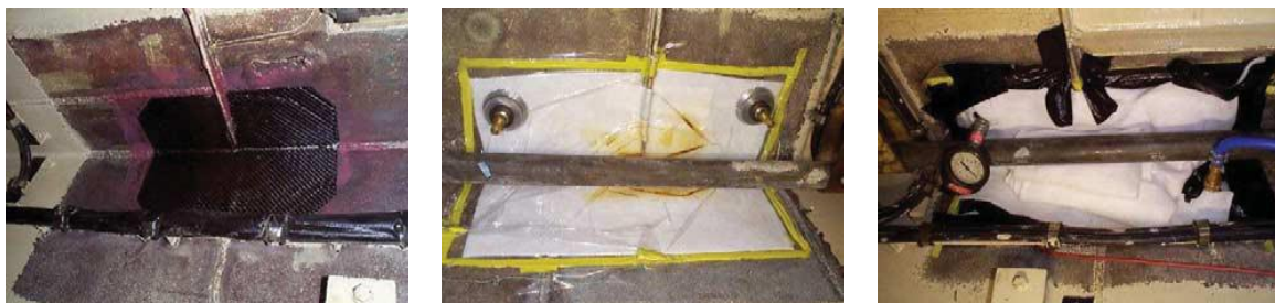
Figure 1.8: Composite patch repairs on lift shafts of Type 42 destroyers.
