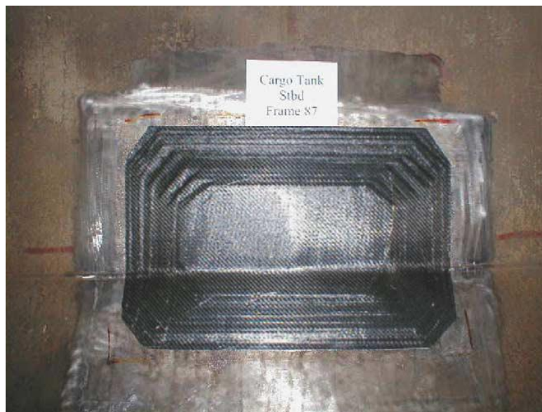
Figure 1.9: Composite patch applied to cargo tank on-board FPSO ( Turton et al 2005 ).
