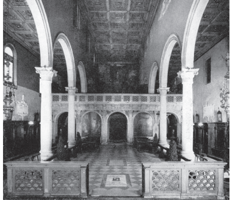
Fig. 14 The tramezzo at San Michelle in Isola, Venice (M. B. HALL, The Ponte in S. Maria Novellae. The problem of the Rood Screen in Italy , in Journal of the Warburg und Courtauld Institute 37, 1974, pl. 38b).
