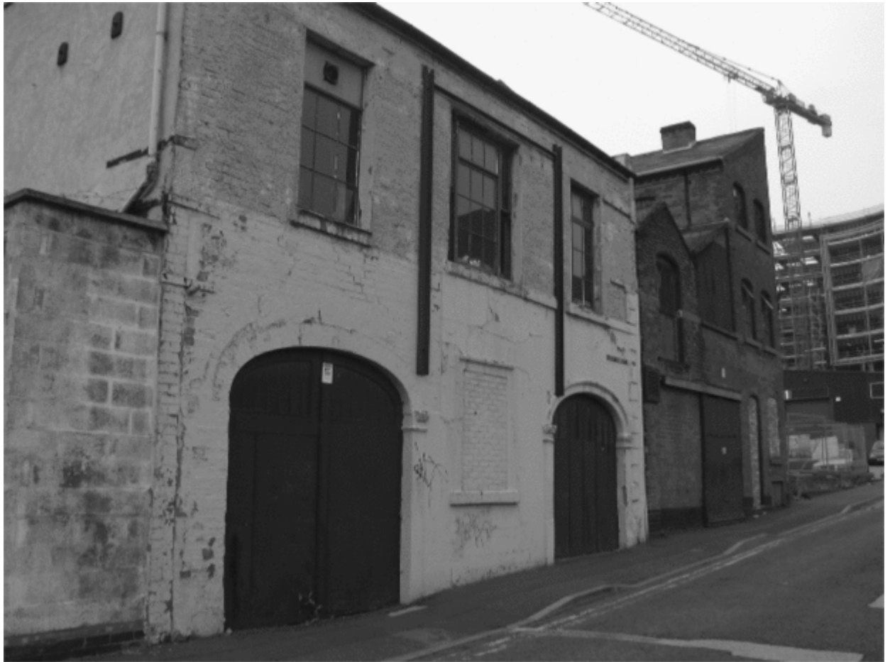
Figure 2. Disused buildings in Grosvenor Street
