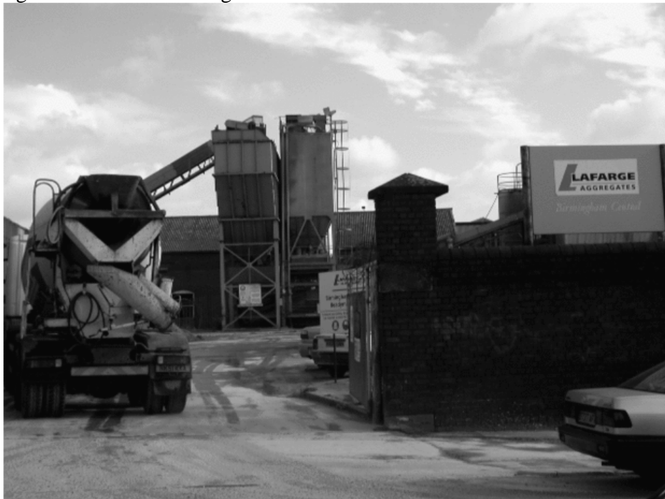
Figure 3. Aggregates crushing in Fazeley Street
