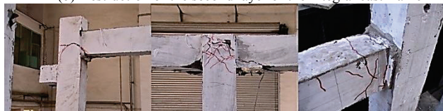
(c) Destruction of the third layer of the integral cast frame
