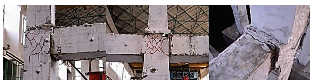
(a) Destruction of the first layer of the integral cast frame
