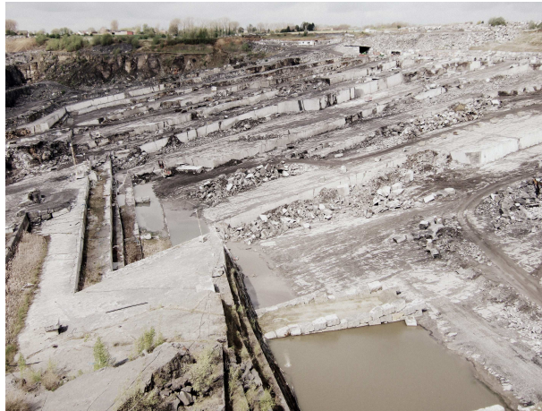
Figure 1: The Neufvilles (Clypot) quarry site (Walloon Region, Belgium). The quarry has a maximal dewatering flow of 2.000.000m^3 per year. The water table dropped from an initial altitude of 70m down to currently 25m . Picture courtesy of Louise Collier.
