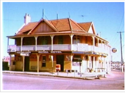
Royal Hotel, Campbelltown before demolition. 1986. (The History Buff)
