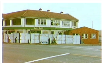
Lacks Hotel Campbelltown about to be demolished in 1984. (The History Buff)
