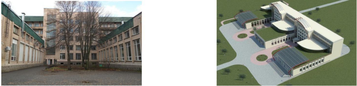
Figure 5.1 Hidrocorpus of Peter the Great St. Petersburg Polytechnic University. Modern look - on the left, Right - the project of reconstruction ( http://www.citywalls.ru )
