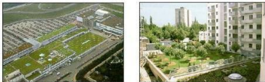
Figure 3.3 Extensive green roof in Germany (left). Intensive green roof in Germany (right) ( http://www.greenroofs.com/Greenroofs101/intro.htm )
