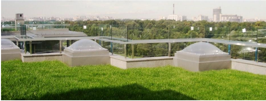
Figure 4.1 Green roof of a residential complex "Diadema"
