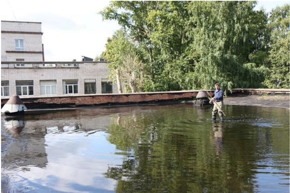
Figure 5.3 View of the Gidrocorpus roof
