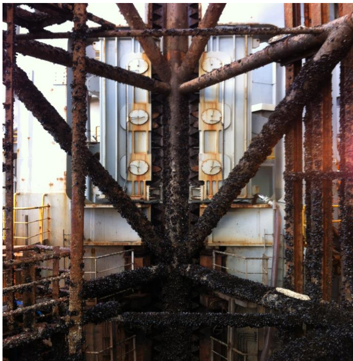
Figure 5. Part of a rigleg and jacking system of the Paragon jack-up rig
