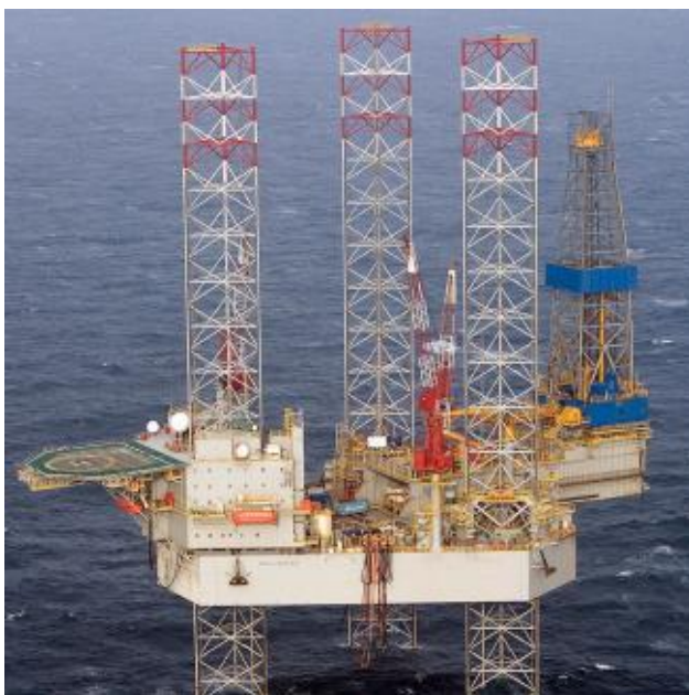
Figure 6. Hans Deul jack-up rig
