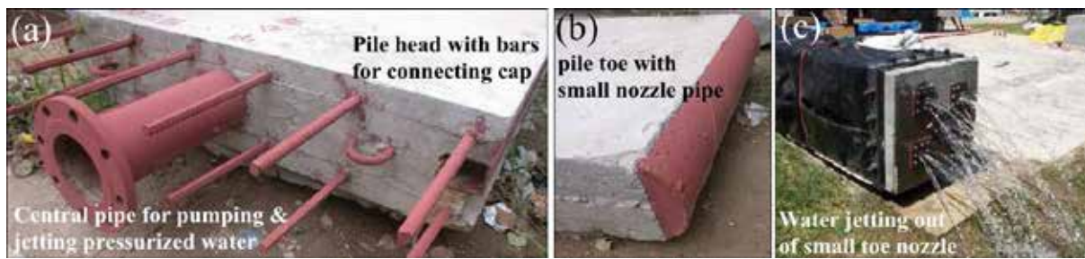
Figure 3: Flexible design of head and toe of precast reinforced concrete piles for jetting and grouting installation
