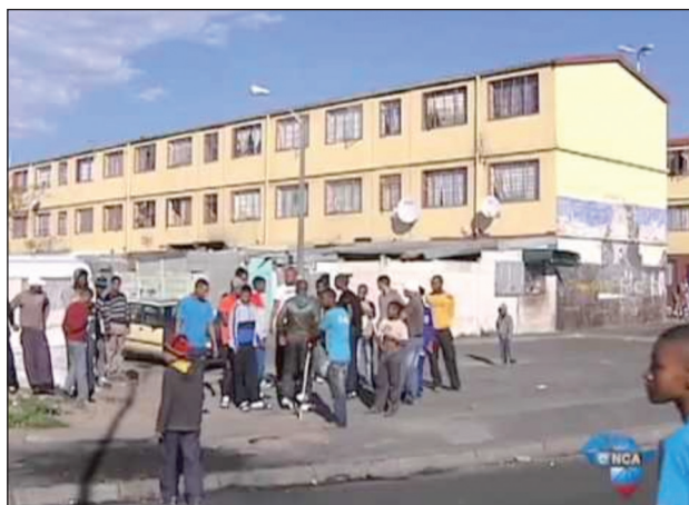
Figure 19. Example of large scale low cost housing (Class #3) found in Manenberg on the Cape Flats, Tongaat near Durban and Zwide near Port Elizabeth.
