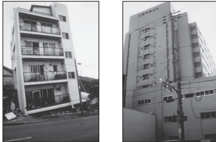
FIGURE 3 (above left). Typical example of building class #8 consisting of ‘reinforced concrete shear wall, without moment resisting frame, medium rise’. Source: EMS98 (op. cit.)
