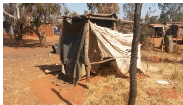
Figure 12. Current Ablution Structure Covered by Plastic Sheeting (Coetsee.et.al., 2014).[1]
