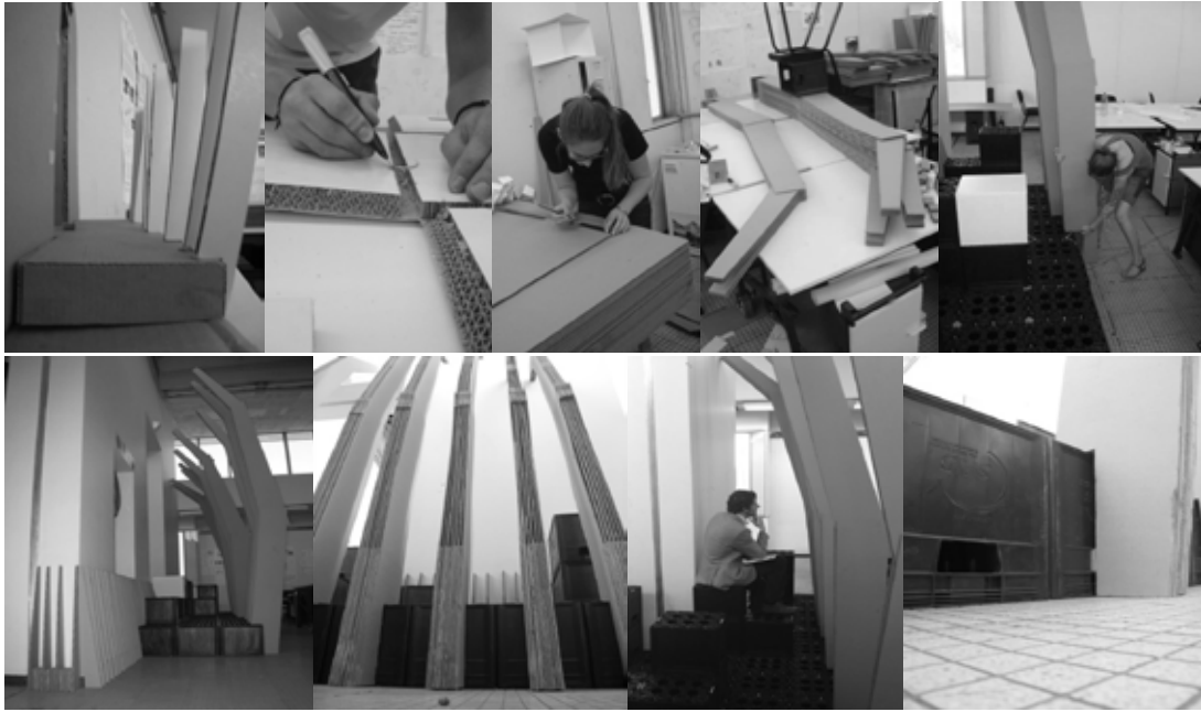
Figure 2 Complete design/build process of Group E: modeling, prototyping and fabrication ( top ); installation, use and evaluation ( bottom ).
