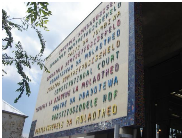
Figure 19: Exterior of the Constitutional Court, Johannesburg, 2007. Photograph by the author.
