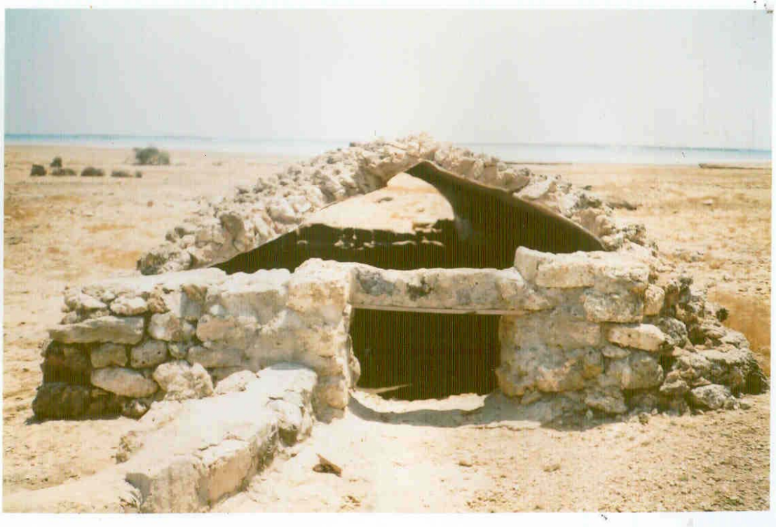
Figure 6.2: Dahlak Islands. A Caged Well (In Dahlak Kebir Island) With The Idea Of Preventing Evaporation
