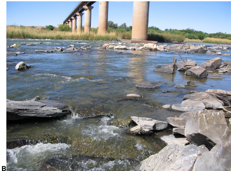
B Fig. 2.7 Satellite view (A) (Google Earth) and photo (B) of Sishen Bridge in the Orange River.
