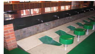
(Left: Fig. 23. Dar-as-Salaam Mosque, Laudium, South Africa, 2002, indicating the individual cellular trays in the ablution area).
