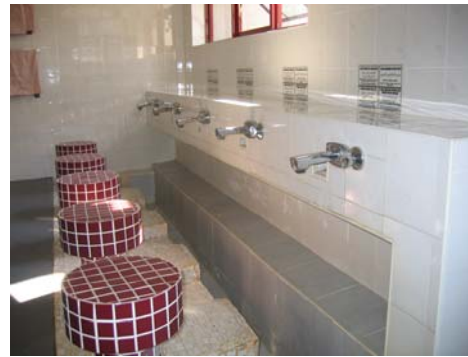
Fig. 2. Mosque survey: Brits Friday Mosque. Illustrating ablution area
