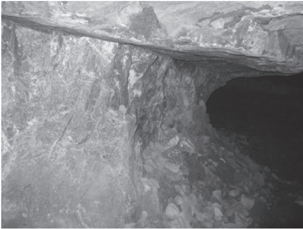
Figure 1—Example of crush pillar deformation behaviour
