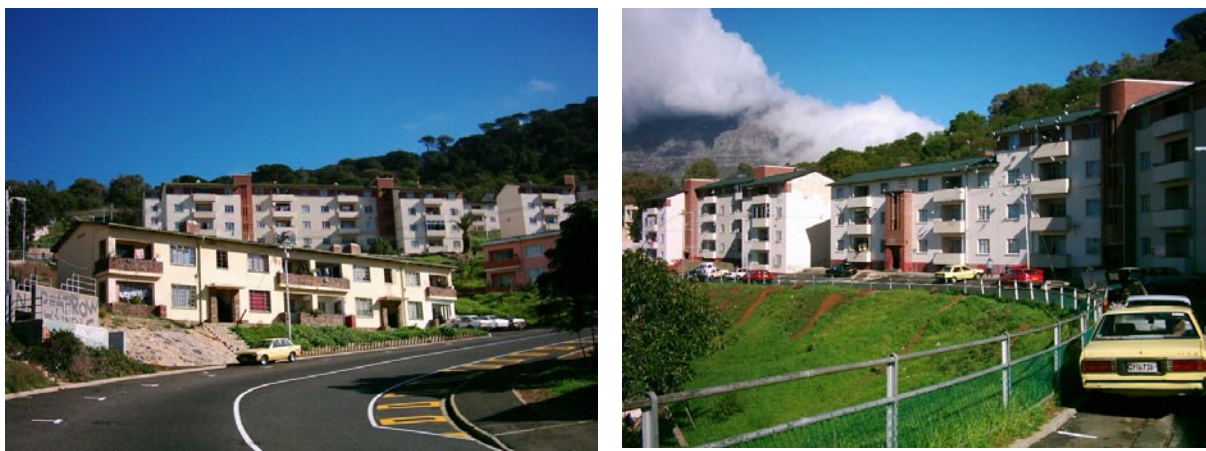
Figure 5 The Schotsche Kloof Flats (photographs by the author 2005).
