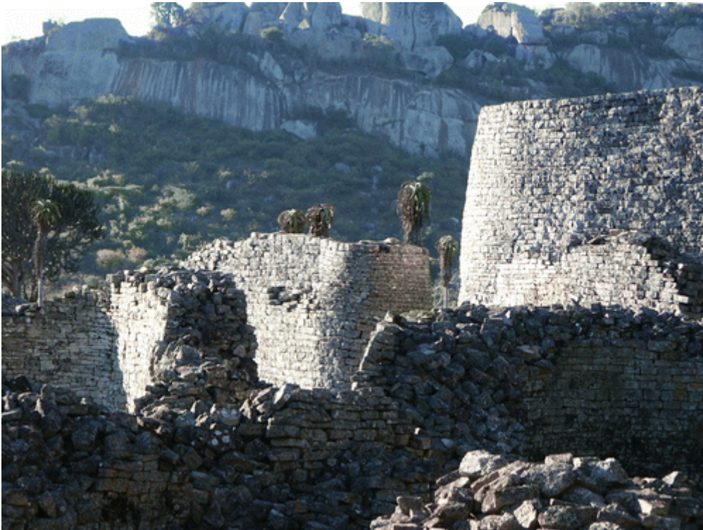
Figure 2. Rounded entrances at Great Zimbabwe. Note the similarities with Jahunda and the neat coursing that belongs to the Q style of walling.
