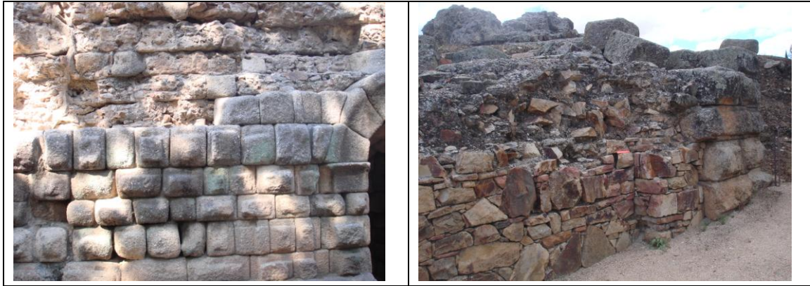
Fig. 2. External wall from the theatre (left) and amphitheatre (right).
