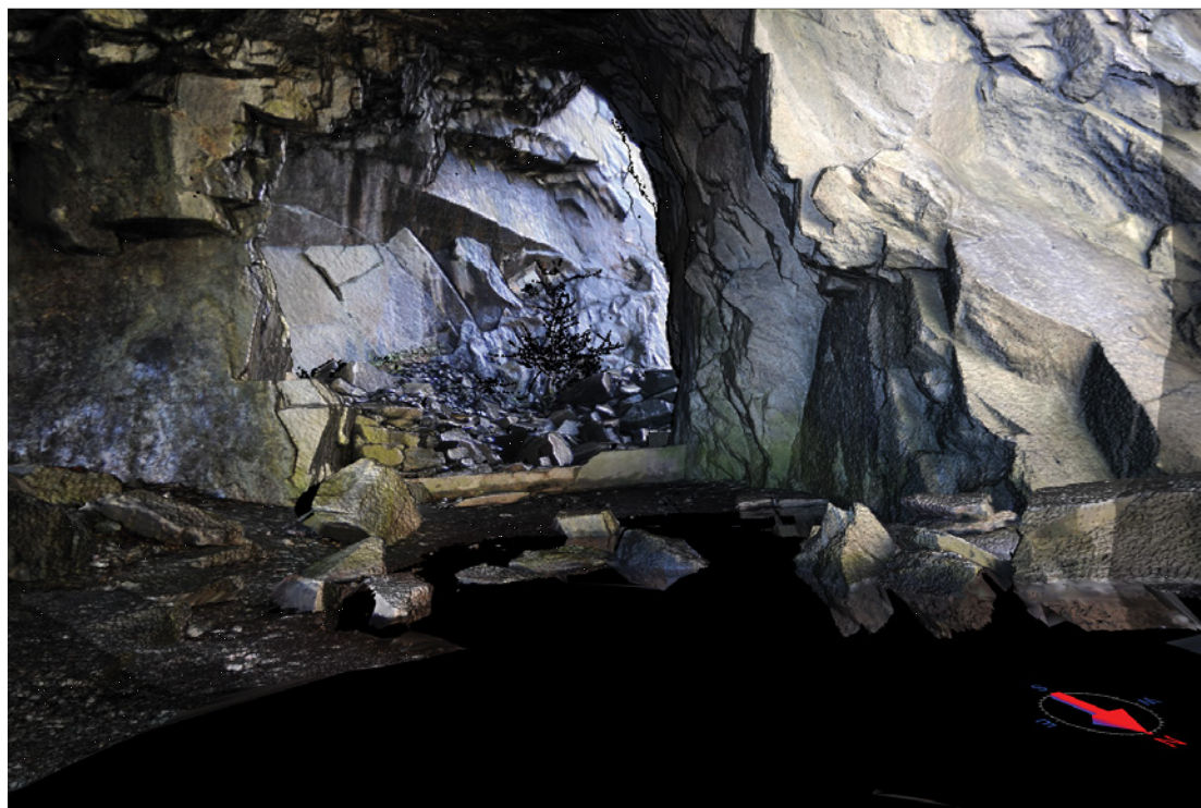
Figure 6.8: 3D photomosaic combined with 3D lidar scan of Hodge Close Quarry (NY 31685 01694). Rocks are part of the Seathwaite Fell Sandstone Formation, Borrowdale Volcanic Group
