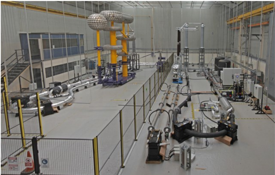
Figure 2-9: Alstom HVDC cable ageing facility, Stafford UK [82].
