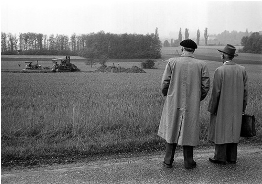
Fig. 13: Geneva officials and CERN staff survey Meyrin as construction of CERN begins.
