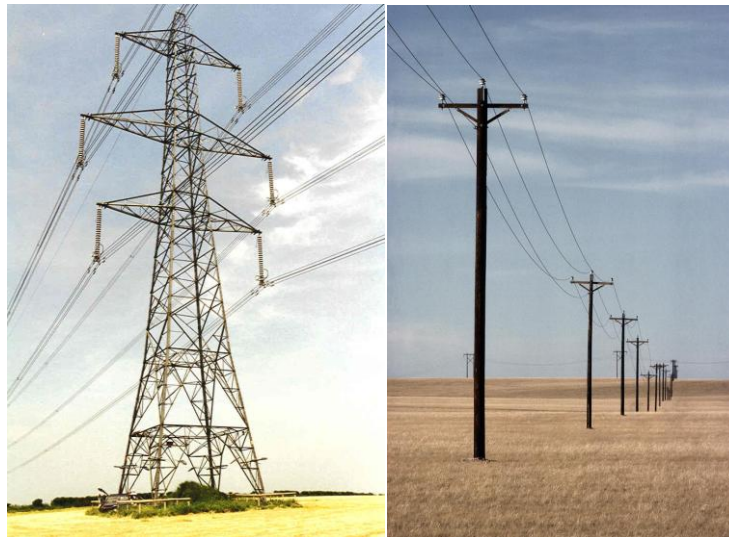
Fig. 1-1: Example of overhead line mounted on metal pylon (left) and wood pole (right)
