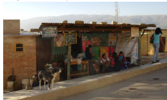
Image 16 Small shop built inside of the house
