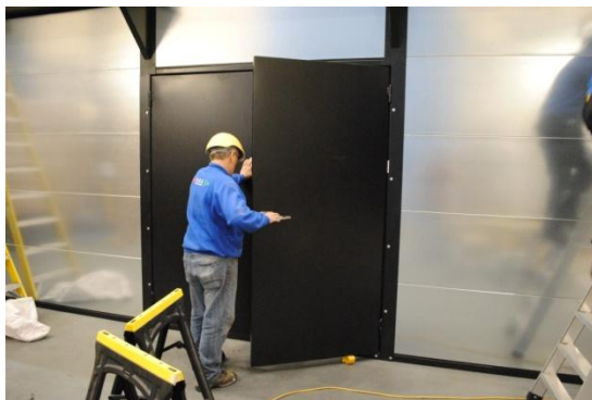
g). installation for the doors
