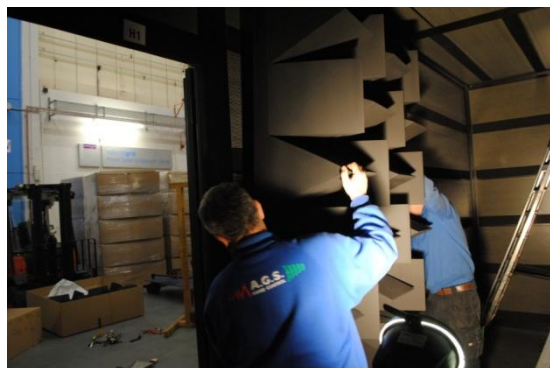
h). attach the wedges
