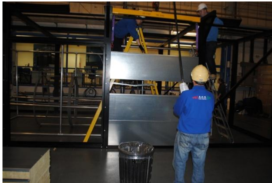
c). fit in panels
