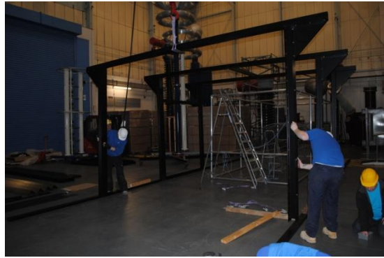
b). installation for the frame
