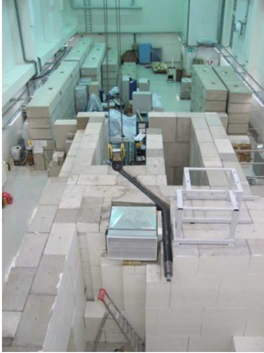
(a) Construction of IGISOL 4 (March 2011).
