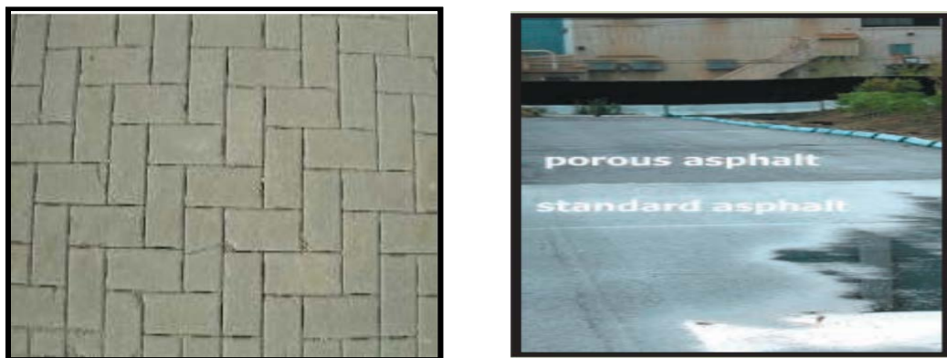
Figure 7 Permeable pavement (left : ((Myers et al., 2007))) Porous pavement (right : (Cahill et al., 2003))
