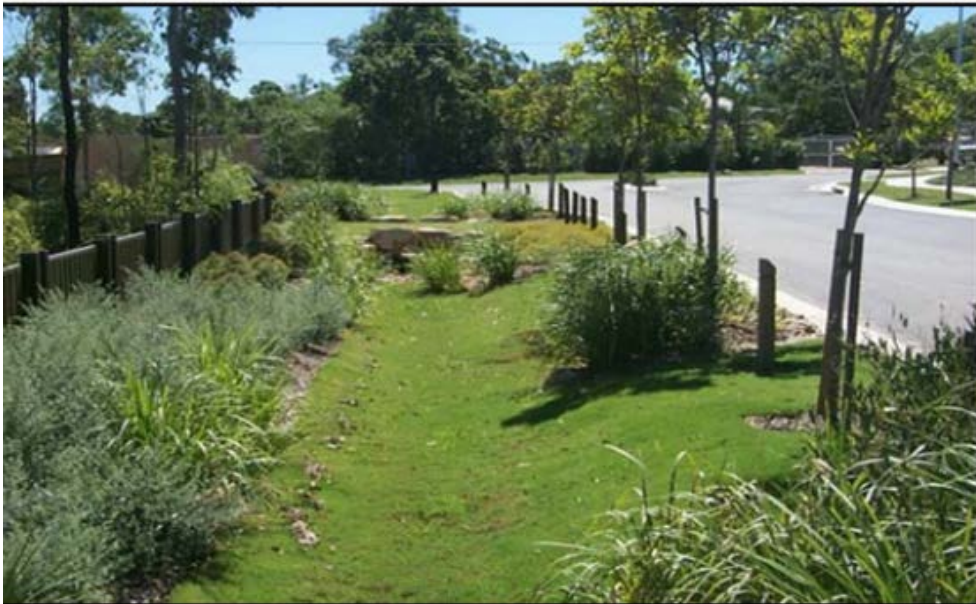
Figure 9 Grass swale used in a residential area in Australia (Wong & Taylor, 2002)
