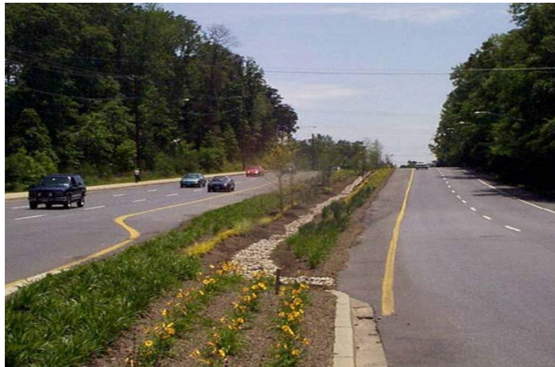
Figure 5 Infiltration trench used in a traffic island (LID, 2010)
