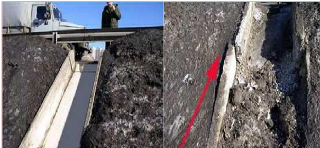
Figure 2.9: Comparison of the performance of FRP composite channel (left) and reinforced concrete channel (right) (Bernard Potyrala, 2011)
