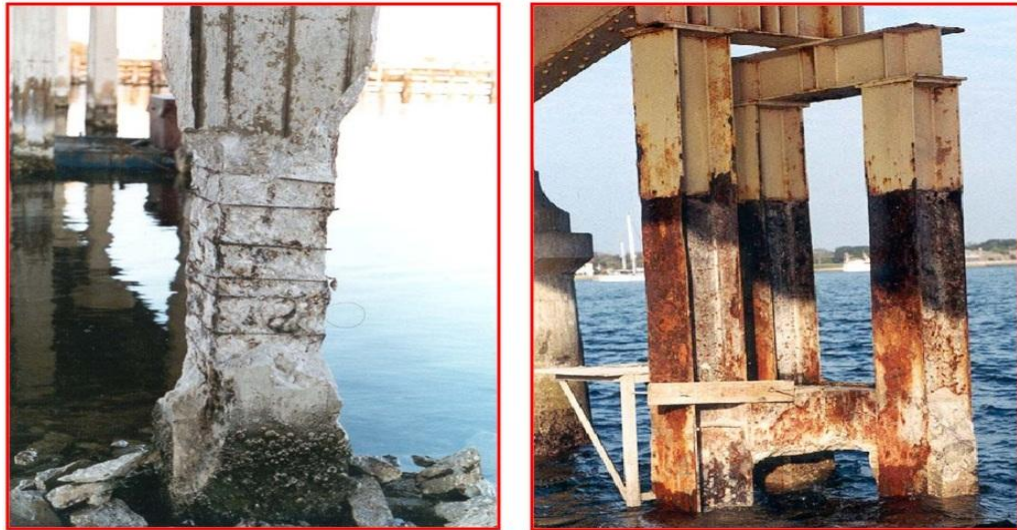
b) Corroded steel piles
