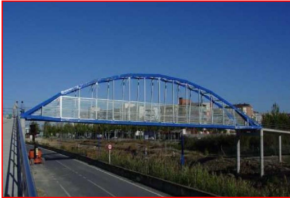
Figure 2.11: General view of the Lleida footbridge (Spain) (Bernard Potyrala, 2011)
