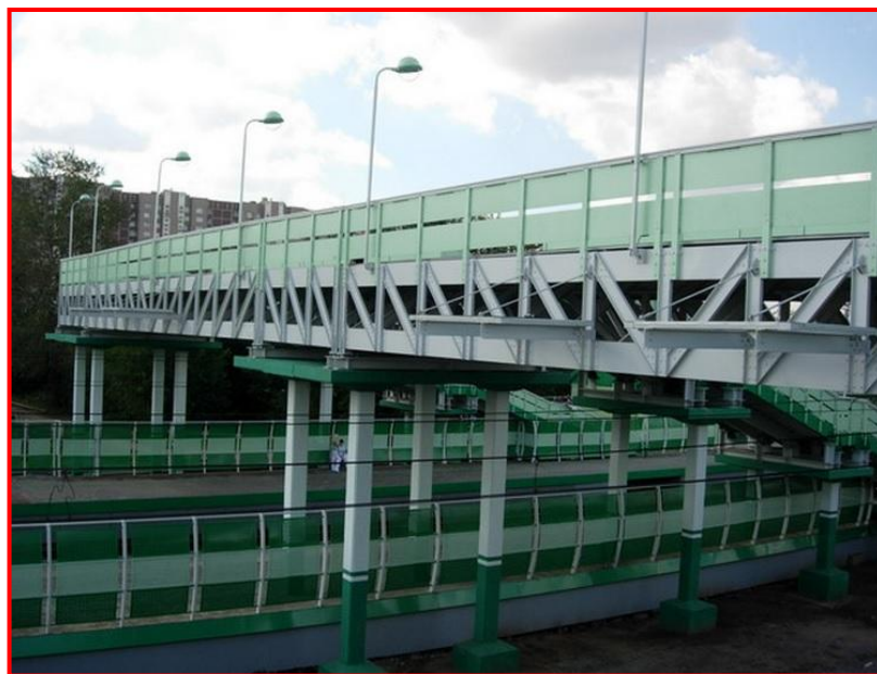
Figure 2.10: FRP composite pedestrian walkway in Russia
