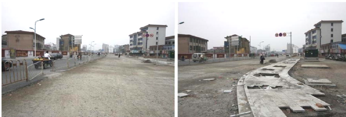
Figure 7.26. The retrofit construction of Chengnan Road in 2006
