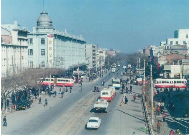
Figure 7.16. Photograph of Dazhi Street in the 1980s
