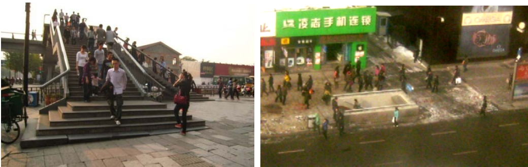
Figure 8.18. The pedestrian bridge at Intersection B in Qingchun Road (left) and the underpass at Intersection J in Dazhi Street (right)
