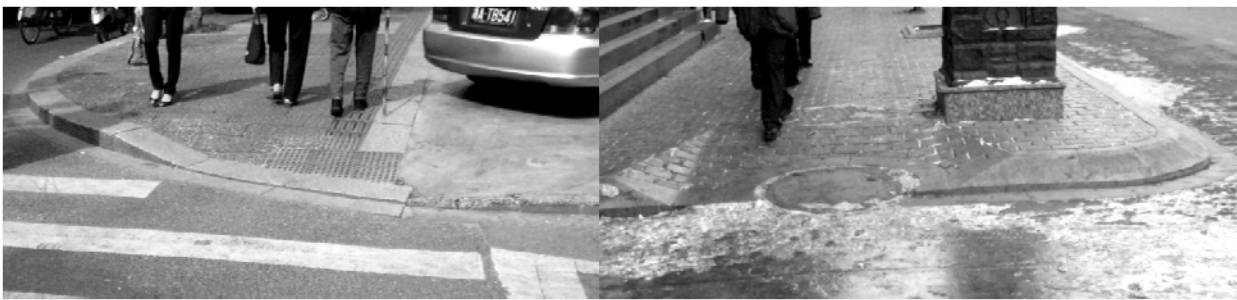
Figure 8.39. The enlarged kerb ramp in Zhongshan Road (left) and the regular kerb ramp in Guogeli Street (right)
