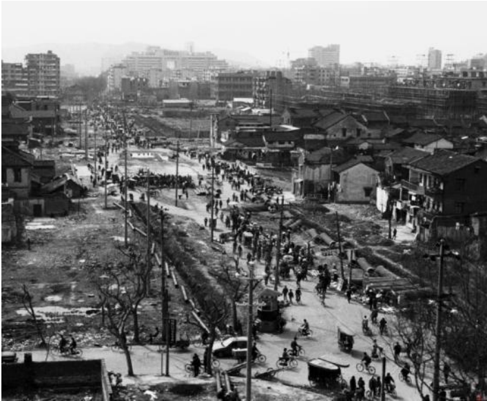
Figure 7.8. The reconstruction of Qingchun Road in 1992
