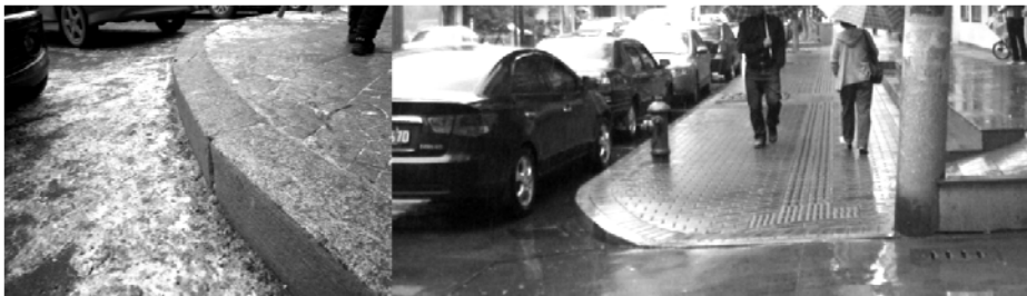
Figure 8.64. The raised and sharp edge of pavement in Manzhouli Street (left) and in Haier Xiang (right)
