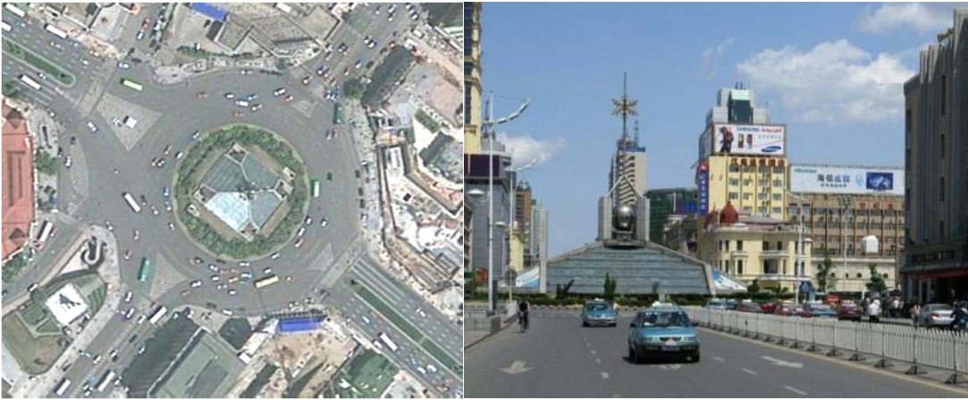
Figure 7.17. The satellite view (left) and the photograph (right) of the roundabout in Dazhi Street
