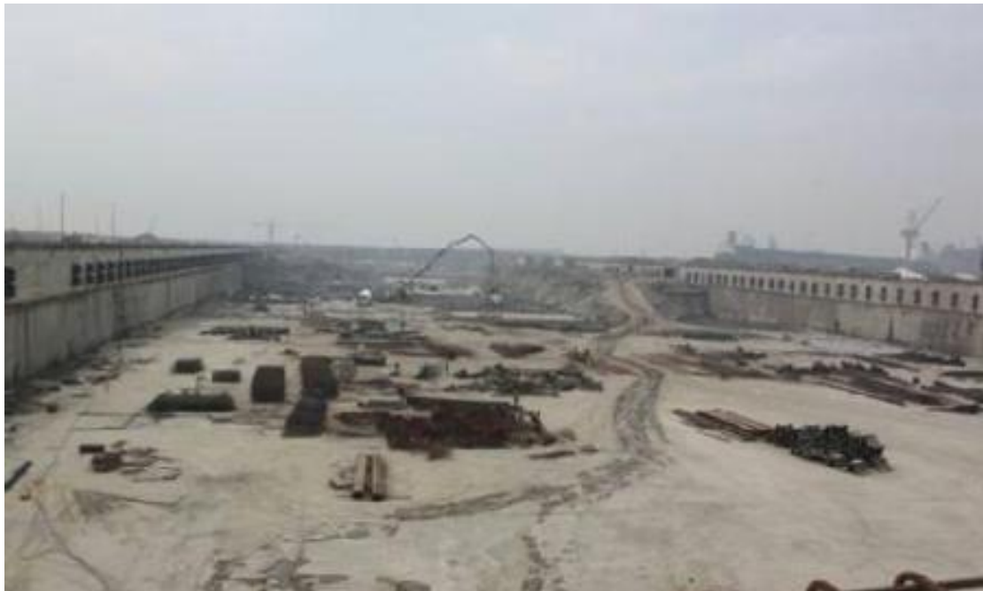
Picture 14: CSG No. 4 Dock for Offshore Engineering under construction in Nov. 2010.
