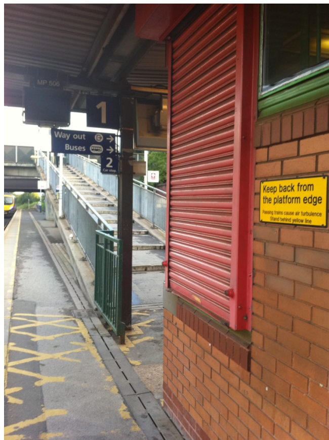
Figure 5.4: Narrow platform and ramp linking the platform to the right-of-way bridge (picture taken by G. Biesek Mar/2011 at Salford Crescent Station)
