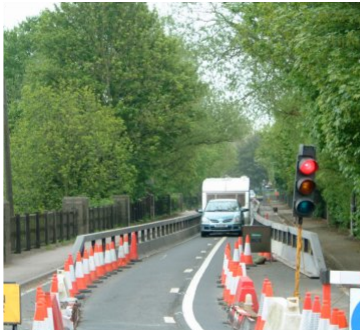
Figure 4.1: The old viaduct during an imposed one-way reversible traffic
