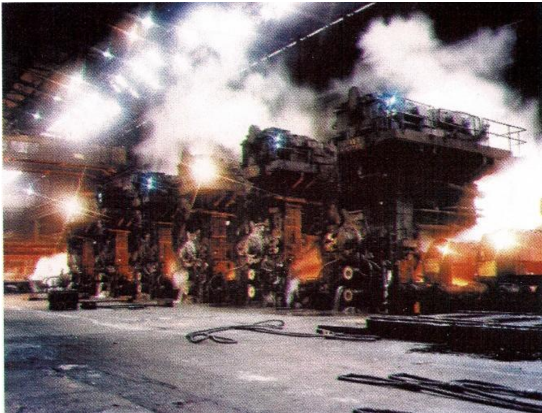
Figure 2.2 Rolling Stands in Operation (Tata steel) [12]
