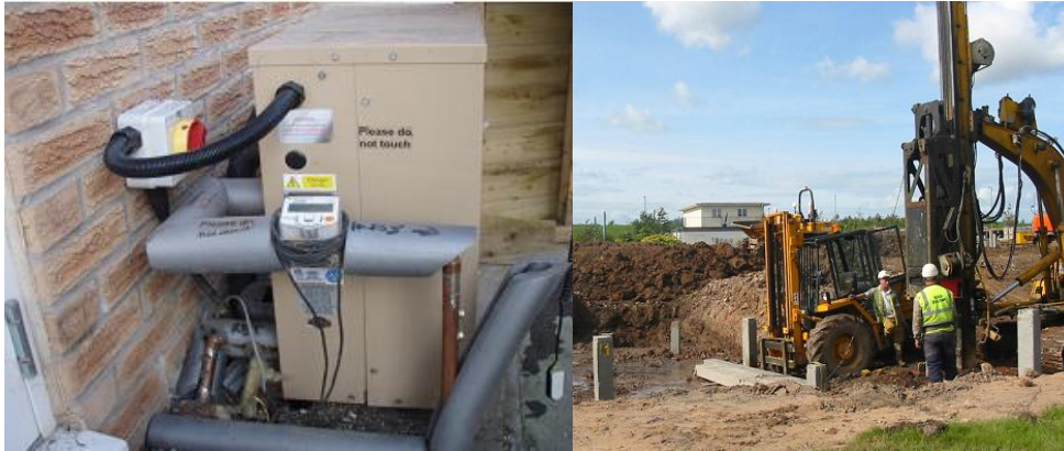
Figure 13.3: GSHP unit (left) and borehole/piling operations (right)
