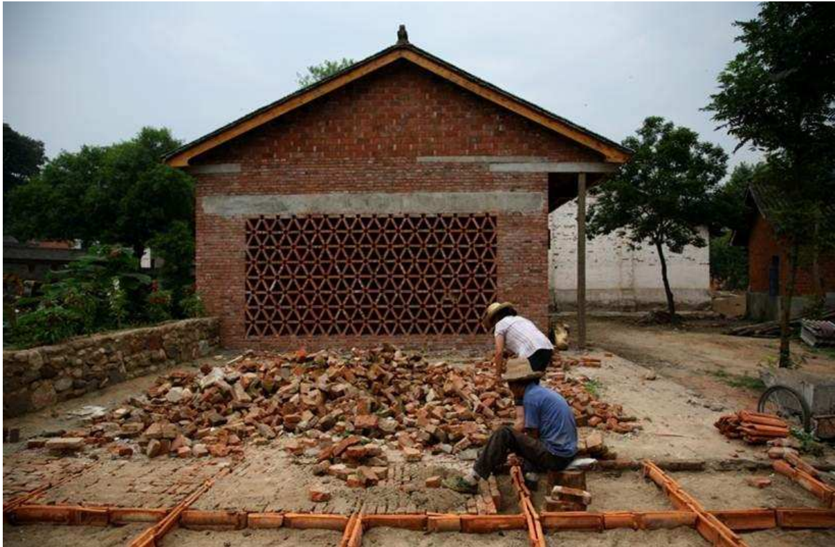
16 Collective construction process on site. Summer 2014
