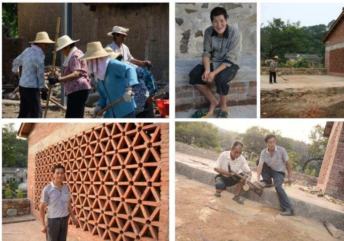
15 The construction team was made up of the remaining women, the disabled, the mason and the carpenter, all from the village. Summer 2014
