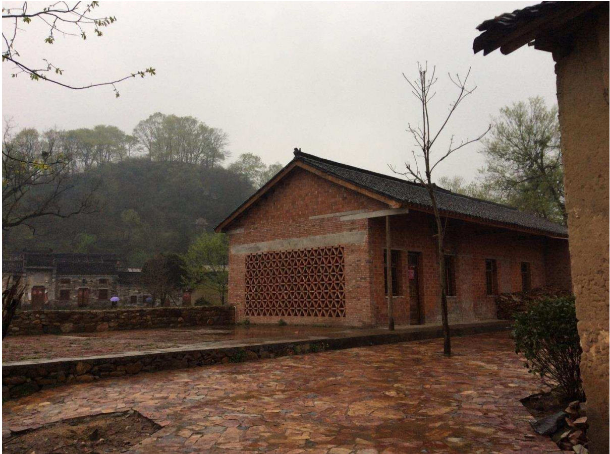
13 A new canteen for the village was transformed from an abandoned building, with its external brick-screen-wall coproduced by the architect and users in a different way from both urban and rural normal practice. One third of the existing volume was demolished in order to leave a ritual visual corridor to assimilate Qi (energy) to the main body of village on the other side of the river. Spring 2015
