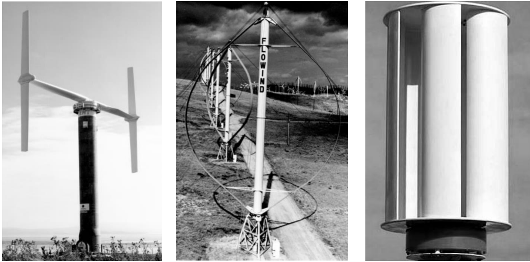
Figure 2:1: H-Type (left), Darrieus Type (middle) and Savonius Type (right) VAWTs [9, 11]
