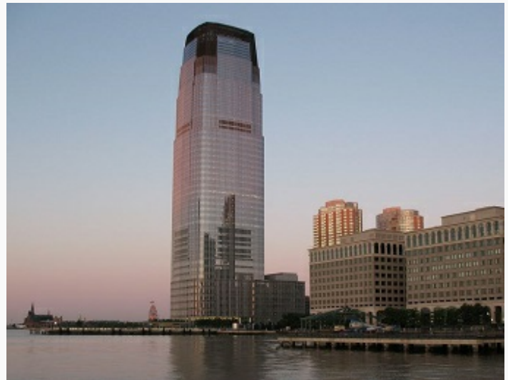
Goldman Sachs building in New Jersey. Credits: click-see (CC BY-SA 2.0)
