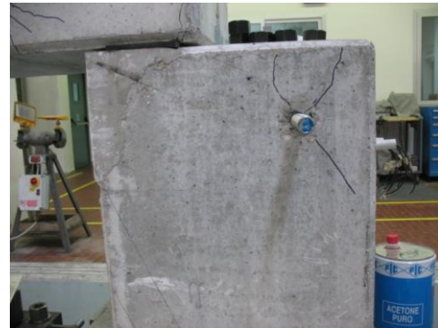
Fig. 14 Cracking pattern around the node 3 East side (test 1)
