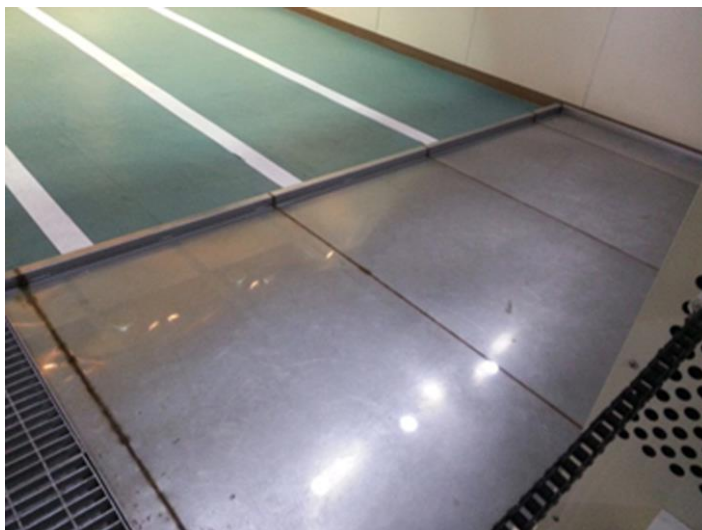
Fig. 11. Gunpowder cleaning gutter in the shooting range.
