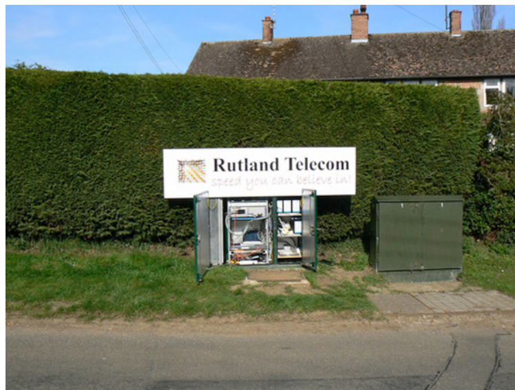
Figure 3.13: Installation of Rutland Telecom FTTC Service in Lyddington
