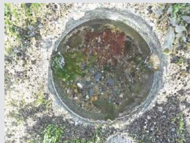
Figure 4 Artificial rock pools installed in an intertidal breakwater in Wales, UK, provided important habitat for marine life and performed a similar function to natural rock pools on nearby rocky shores (Evans et al. , 2016). © Ally Evans.
