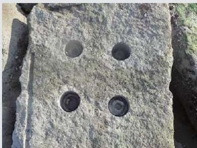
Figure 4 Artificial rock pools installed in an intertidal breakwater in Wales, UK, provided important habitat for marine life and performed a similar function to natural rock pools on nearby rocky shores (Evans et al. , 2016). © Ally Evans.
