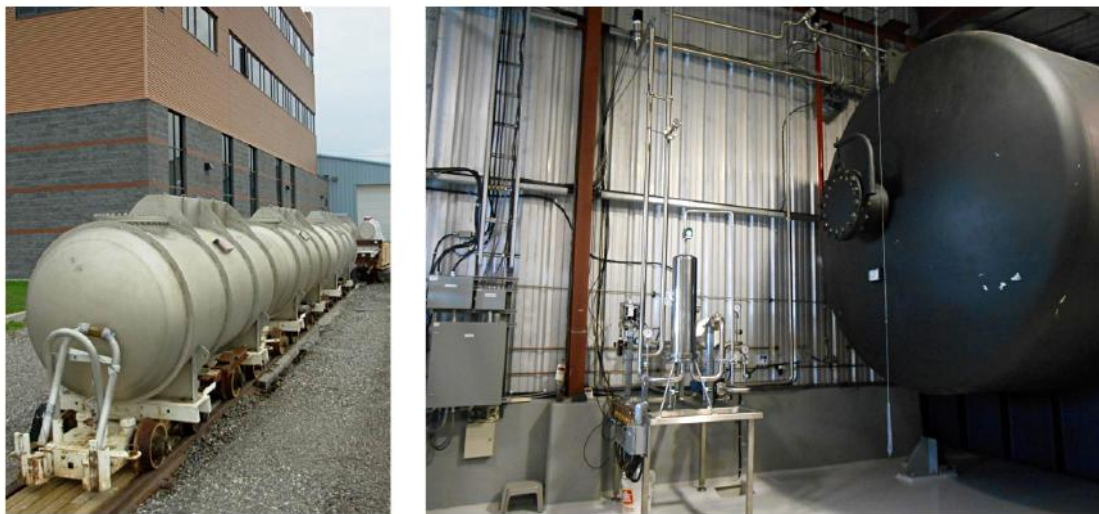
FIGURE 3.17: The surface rail tankers (left) used to transport the LAB from the SNOLAB surface transfer facility (right).
