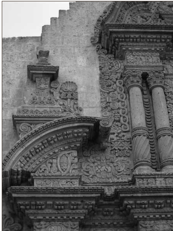
10.3 Central section of the façade of the Church of Santiago, Arequipa. (Photograph and copyright, the author)
