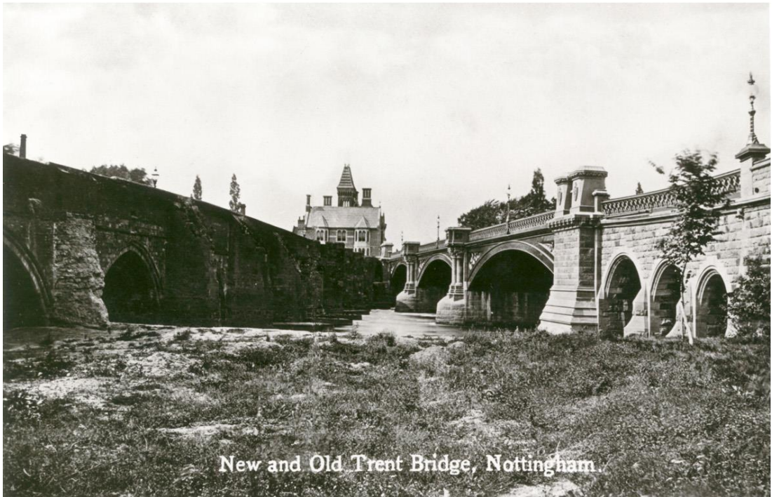
Figure 1 a) Epigraphic markings on Trent Bridge b) The Hethbeth Bridge (left) and Trent Bridge (right), c.1870 (Beckett, 1997)
