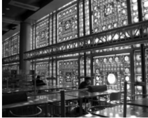
Figure 1. AWI kinetic façade system.
