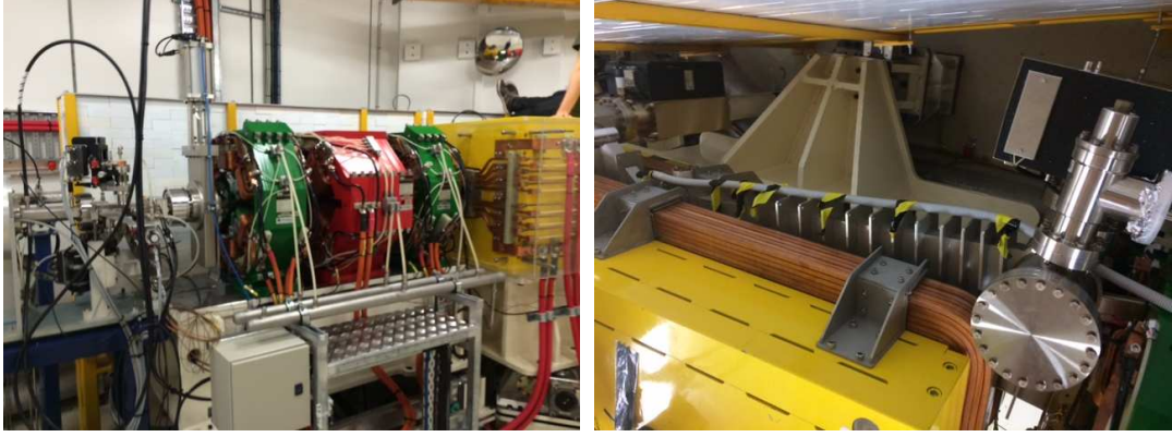
(a) Storage Ring scrapers (far left), Beam Loss Monitors behind dipole (far right). (b) Optical fiber installed in the outer side of the bending magnet, beam from left to right (top view).
