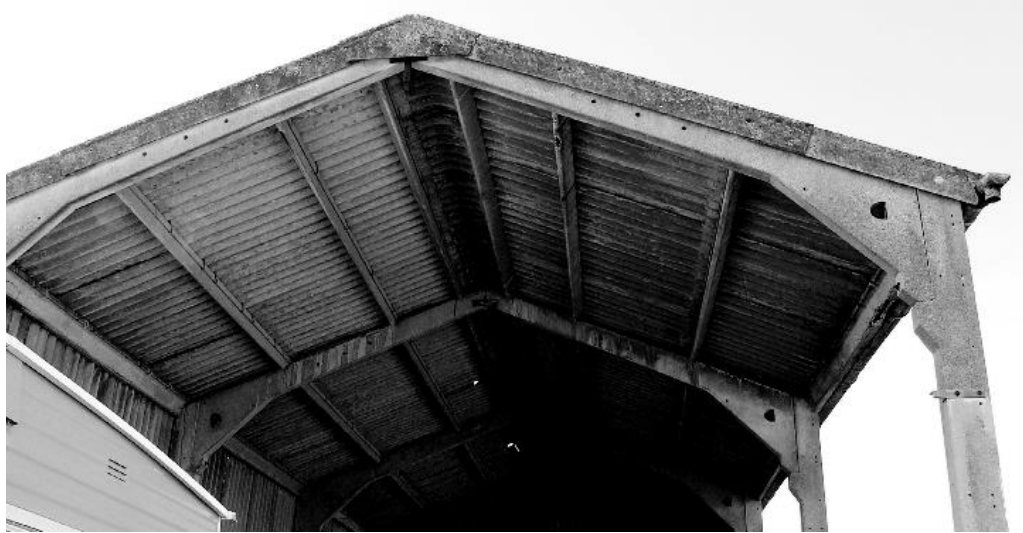
FIGURE 2.73. Demountable concrete frame design 177
