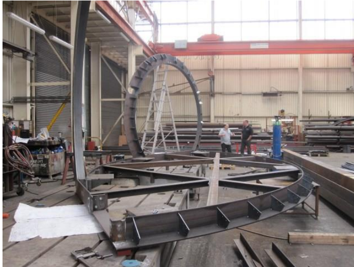
FIGURE 4. 88. The steel foundation being fabricated in Nottingham 87
