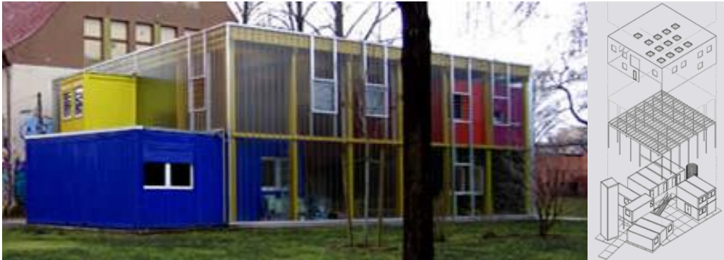
FIGURE 2.71. - 2.72. From left to right: The “Container Village” with an industrial glass shell; The architectural drawing of the design 172
