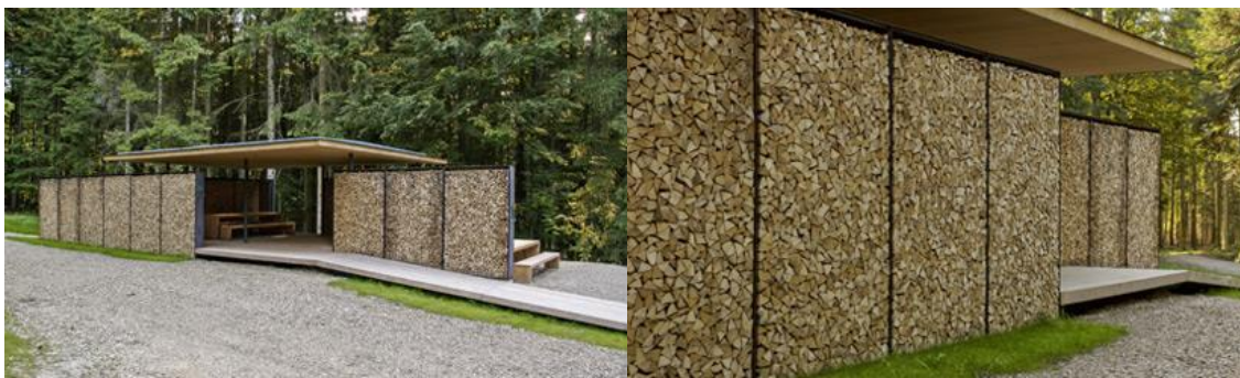
FIGURE 2.82 - 2.83. Waldpavilion Gulpwald, Willisau; Gabion walls constructed from steel and woods 192
