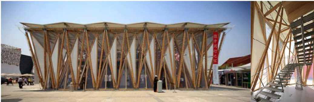
FIGURE 2.39. - 2.40. German-Chinese House, Shanghai, China; An inside view of the pavilion 126
