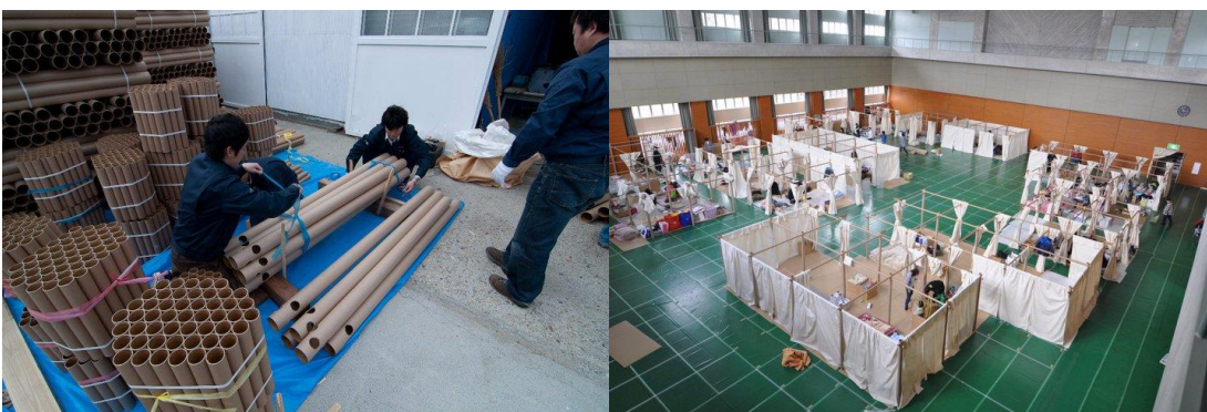
FIGURE 3. 8. - FIGURE 3. 9. Paper tubes in transportation; Paper Partition System in a stadium 78
