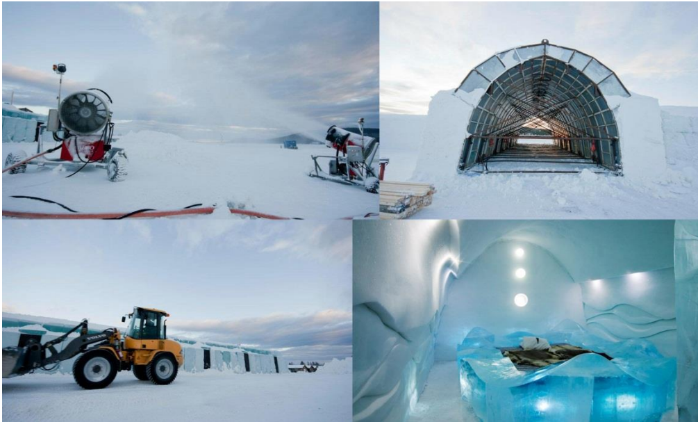
FIGURE 2.85 - 2.88. Snow gun making snow; Snow on the steel forms; Transporting ice-blocks; 196 Art Suite 302 197
