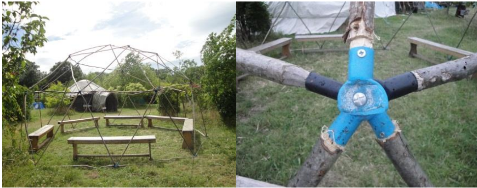
FIGURE 3. – FIGURE 4. The geodesic dome; A detailed view of the structure
