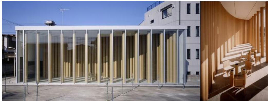
FIGURE 2.46-2.47. Miyake Design Studio Gallery-Shibuya, Tokyo, Japan, 1994; The Interior Design of the Miyake Design Studio Gallery-Shibuya 132
