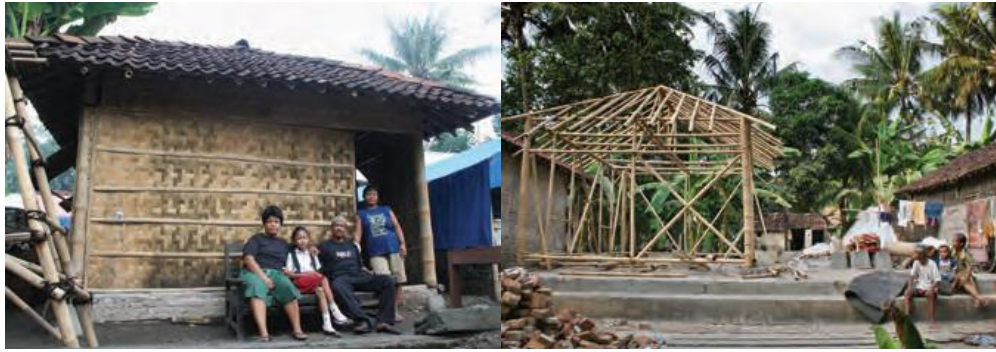
FIGURE 2.37. - 2.38. A completed transitional shelter built through cash grants; A transitional bamboo shelter built on the site of a destroyed house 123
