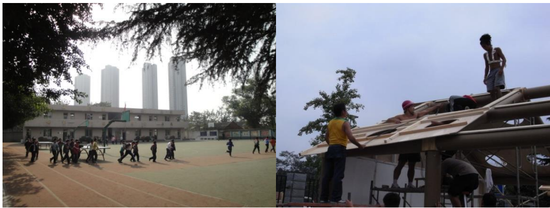
FIGURE 4.31. - FIGURE 4. 32. A view of the surrounding environment; Volunteers working on the building roof 36
