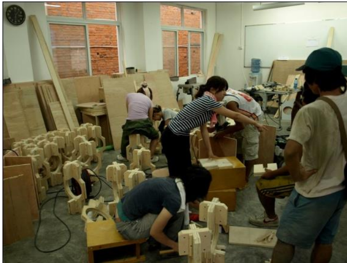
FIGURE 4. 23. A classroom in the concrete building was used as a workshop to store materials and construct small joints 19
