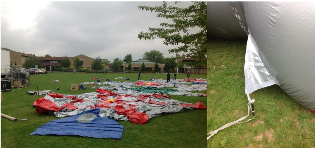
FIGURE 4. 65. - FIGURE 4. 66. The team prepares the structure before inflation; Metal pegs are used to tie the structure to the ground
