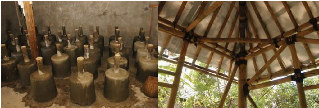
FIGURE 2.35. - 2.36. Foundation pads cast with bamboo connection; Bamboo constructed roof 121
