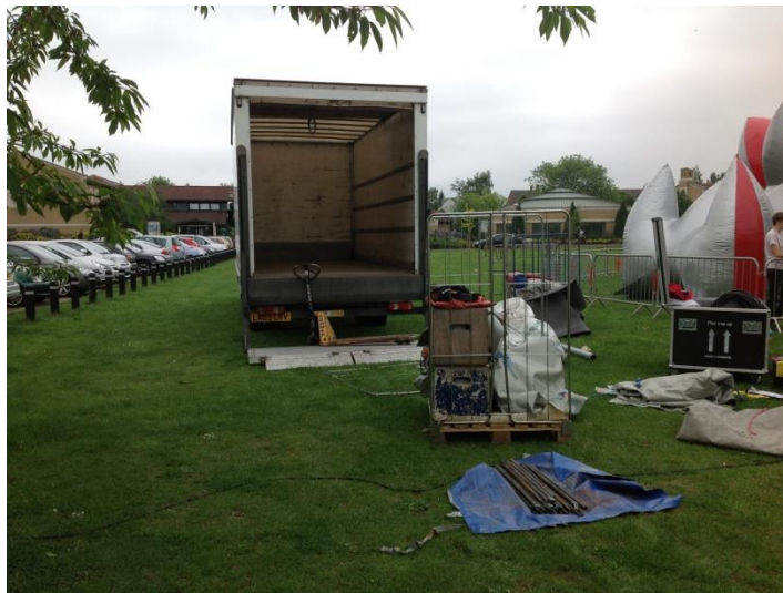
FIGURE 4. 62. A white van was used to transport the whole structure and equipment
