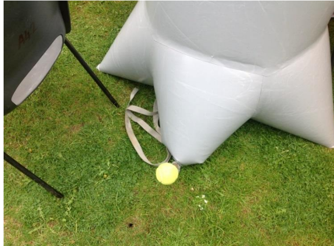
FIGURE 4. 84. A baseball is used on the metal peg to protect the structure
