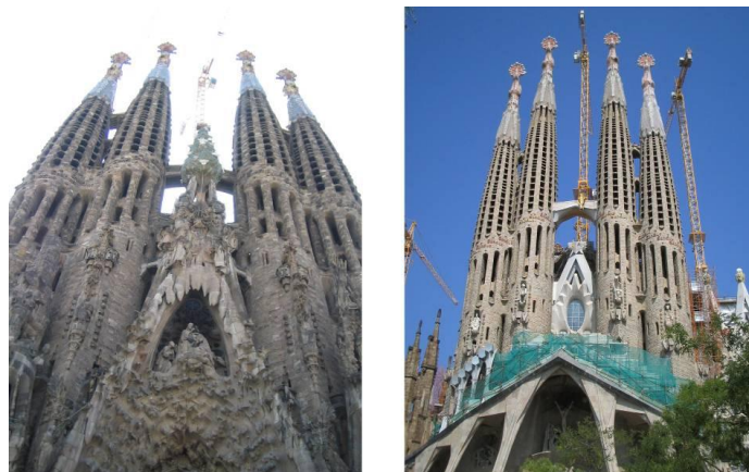
Figure 2.10: The fluidity and plasticity of Gaudi's early designs for the Sagrada Familia church can be seen in the Nativity Façade (left) compared to the Passion façade (right) which utilises ruled surface geometry; a technique Gaudi established in his lifetime.
