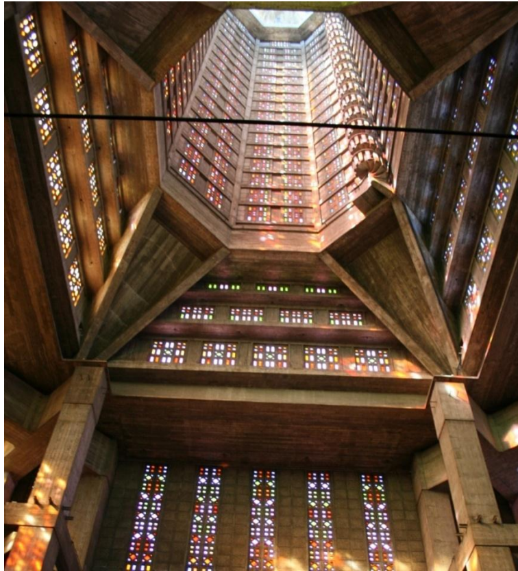
Figure 6.15: Church of St Joseph at Le Havre. Perret adds structure at the corners of the beams as a method of ending the columns.
