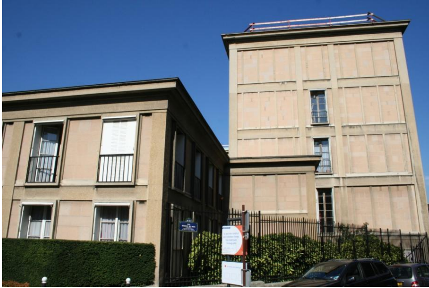
Figure 6.9: The Mobilier National demonstrates the tall and thin windows spanning floor to floor that Perret regularly used. It also shows the secondary columns punctuating the blank façades.
