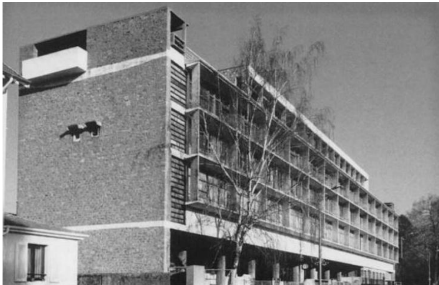
Figure 5.8: St-Dié Factory by Le Corbusier. The elevation treatment and use of pilotis bears a strong resemblance to Stirling's thesis project. Image credit: Gans (2006, p.90).
