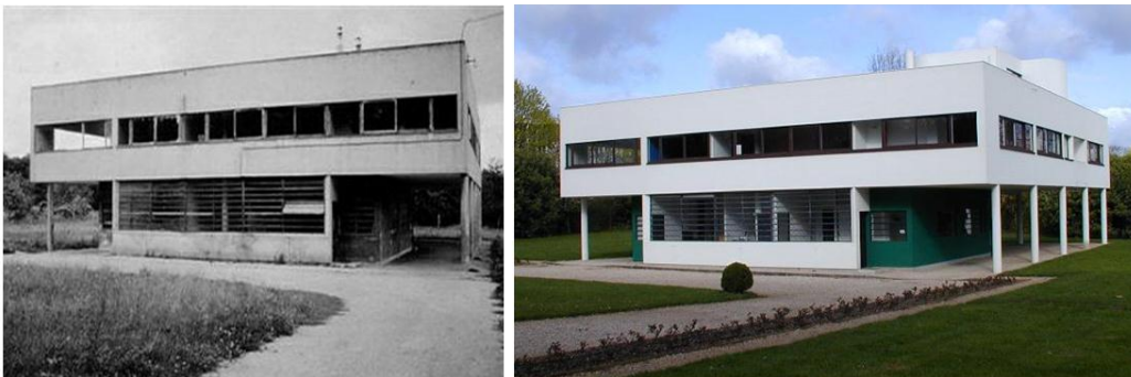
Figure 2.4: Le Corbusier's Villa Savoye in a damaged state (left) and the current building following numerous restoration efforts (right). Left image credit: Mostafavi and Leatherbarrow (1993, p.8), right image credit: cambridge2000.com.
