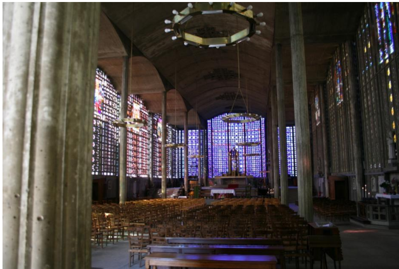
Figure 6.5: Interior of the Church of Notre Dame du Raincy. The stained glass windows are all based on standard dimensions designed by Perret.
