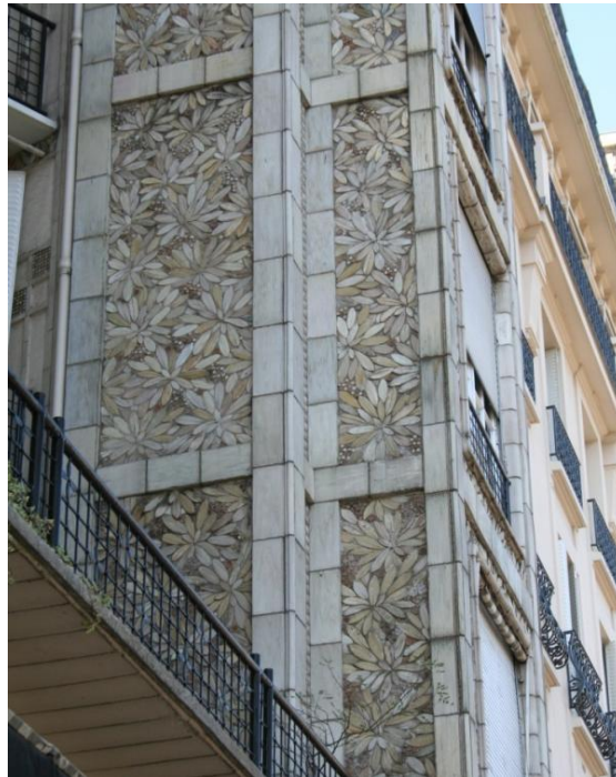
Figure 6.3: Ceramic tiles designed by Alexandre Bigot on Perret's rue Franklin apartment scheme. The leaf pattern is used to show non structural elements whereas the plain tiles indicate the concrete frame.
