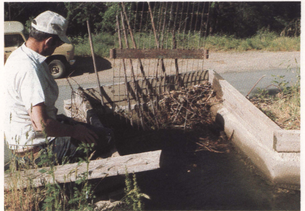
Beaver interfered with crop irrigation by plugging this headgate with sticks and mud.
