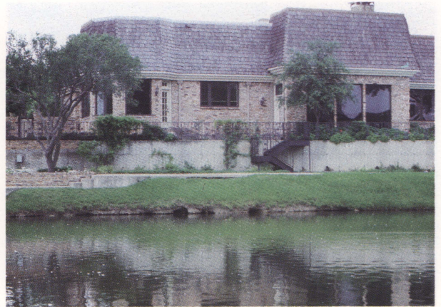
Beaver tunnels under walkways and houses, as shown here, can cause major structural damage if the tunnels collapse.
