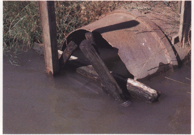
Conibear traps are especially effective where beaver travel through culverts and in shallow runs.
